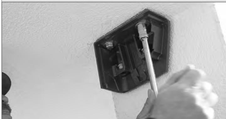
Once the brackets are aligned, tighten the fastener according to the fastener manufacturer's instructions.
