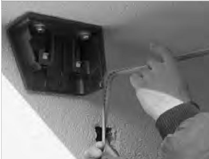
Insert eccentric washers (see Fig. small) in brackets (2 pcs. per side) and attach brackets. Do not fully tighten the fasteners yet. Align brackets (eccentric washers in the brackets allow adjustment of +/- 5 mm in each direction). (see also technical data for bracket attachment).
