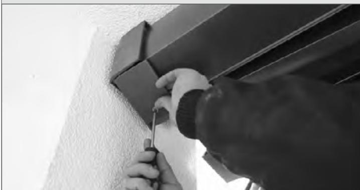
Attach the two covers from below using the supplied fastening screws (2 pieces M 6 x 20 DIN 7991 A2). It may be advisable to extend the awning by approx. 5 cm for this purpose (see Fig.).
