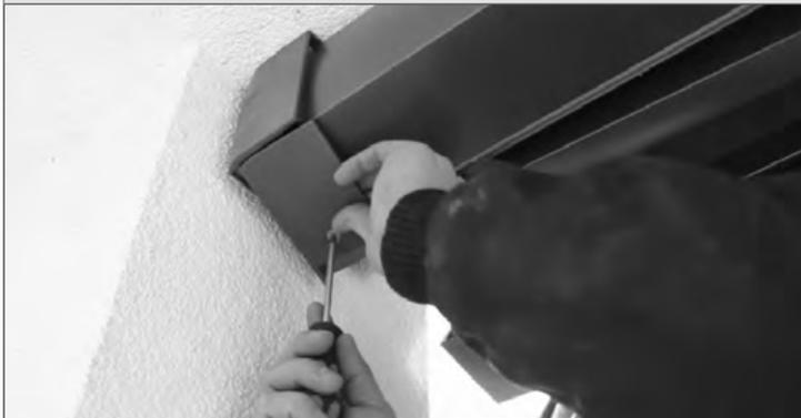
Extend awning approx. 5 cm and remove bracket covers (2 pieces M 6 x 20 DIN 7991 A2).
