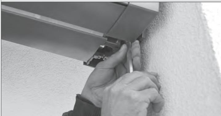
Once the awning is engaged and the brackets are aligned, the awning must be secured with the locking screws before further operation. To do this, tighten the supplied screws „crosswise“ (2 pieces per bracket, M 12 x 45, recommended torque 50 Nm). The locking screws are fully screwed in when the awning can no longer be lifted in the console (see Fig.).
